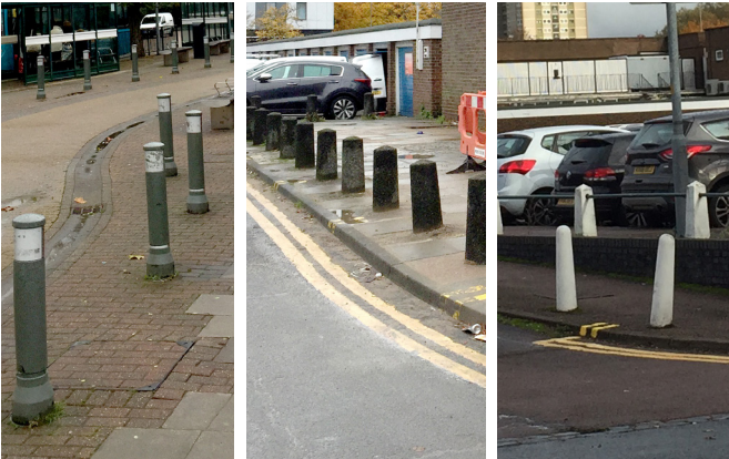
Examples of disparate, aged or damaged bollards that should be removed to avoid visual clutter.
